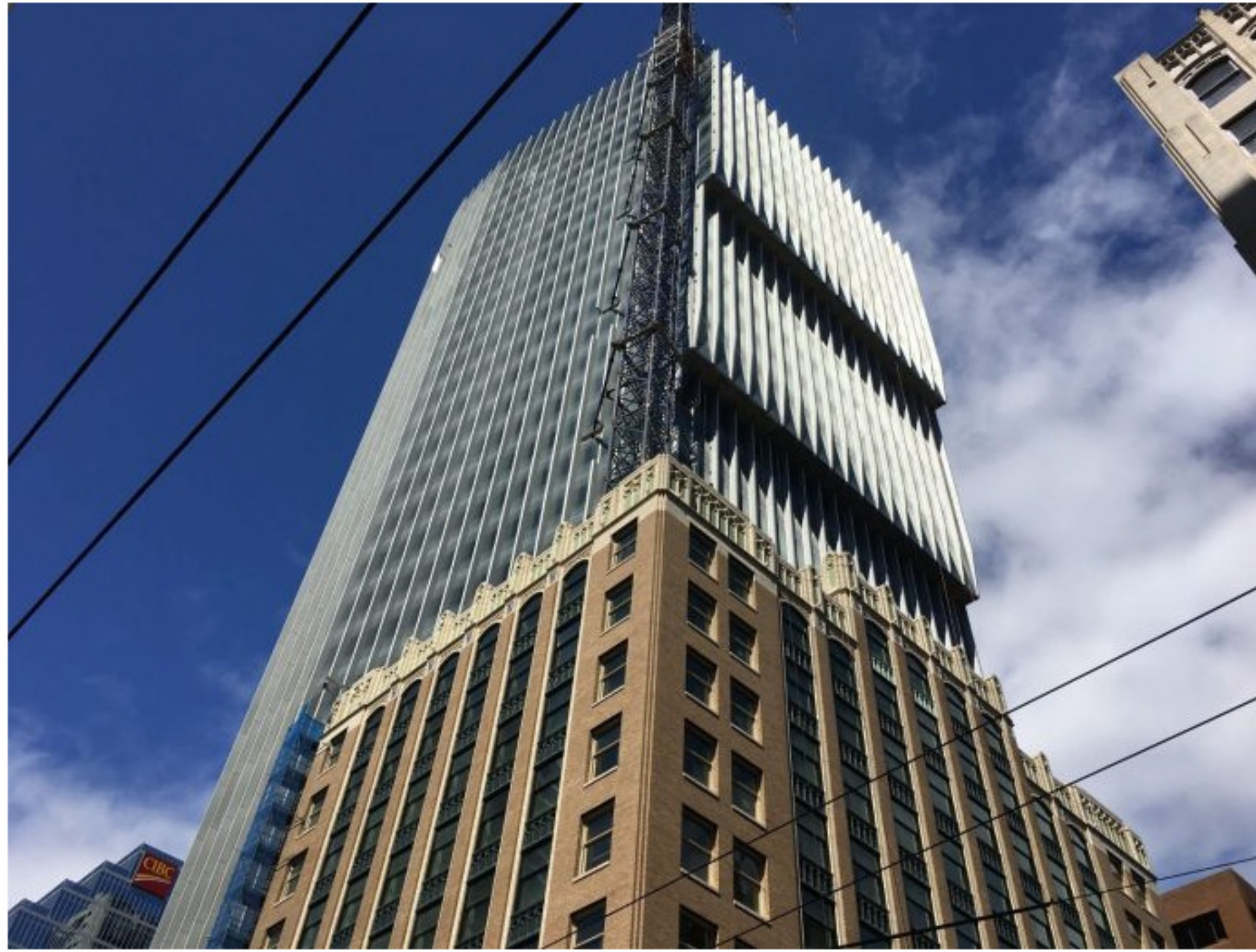
The Exchange office tower under construction in downtown Vancouver.
